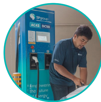
Electric vehicle charging
