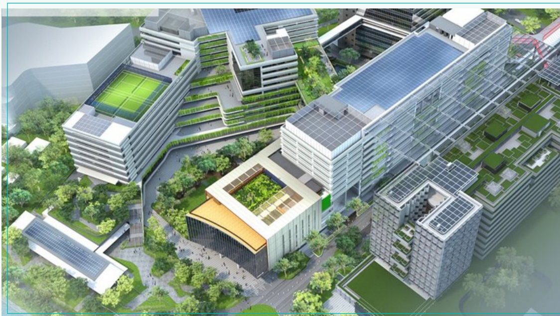
Singapore's largest private microgrid at Singapore Institute of Technology Photo credit: Singapore Institute of Technology
