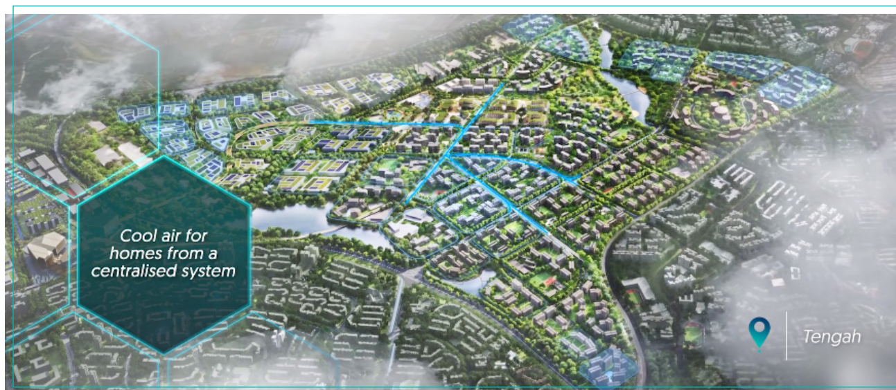
The first large-scale residential district cooling system in Tengah
