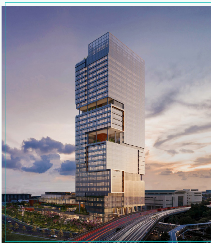
Labrador Tower - achieved Green Mark Platinum Super Low Energy (SLE) certification in June 2022
