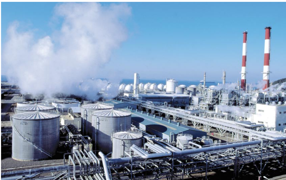
The Seosan industrial utilities complex continued to provide reliable services to Samsung Total during the year.
