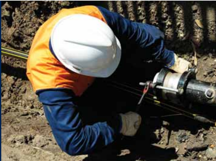
Installing the gas distribution network in western Victoria
