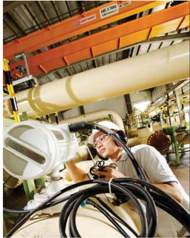
The ultrasonic meter measures natural gas volumes
