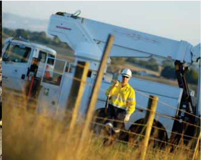
Warragul workers on an electricity distribution job
