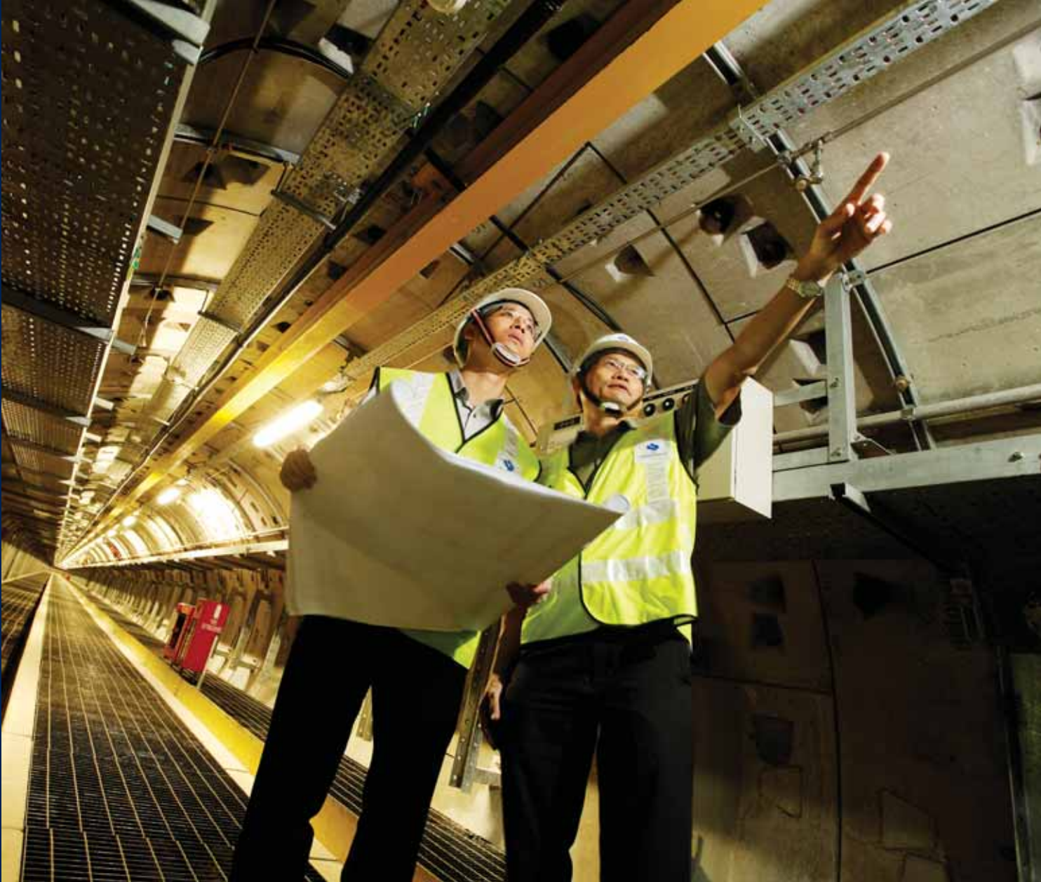
Cable tunnels being constructed for the installation of transmission cables
