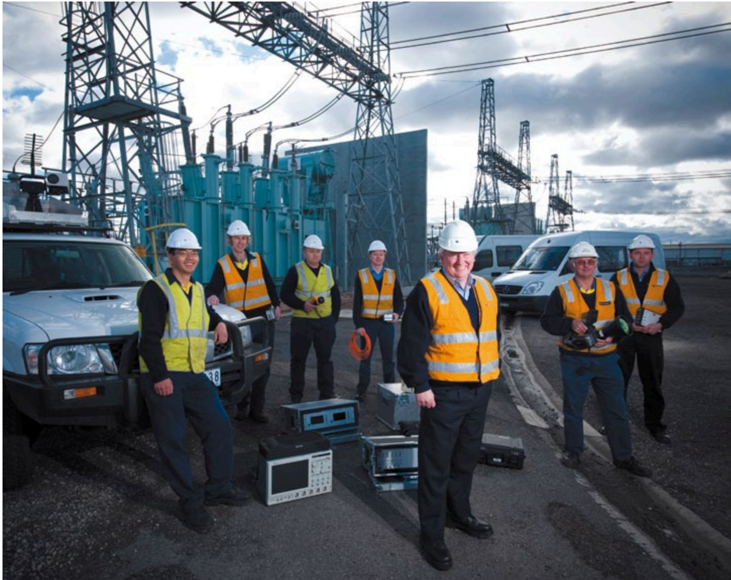
The Condition Monitoring team identifies potential network failures before they occur.
