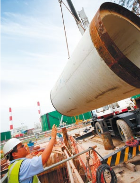
PowerGas continues to renew and reinforce gas pipelines.
