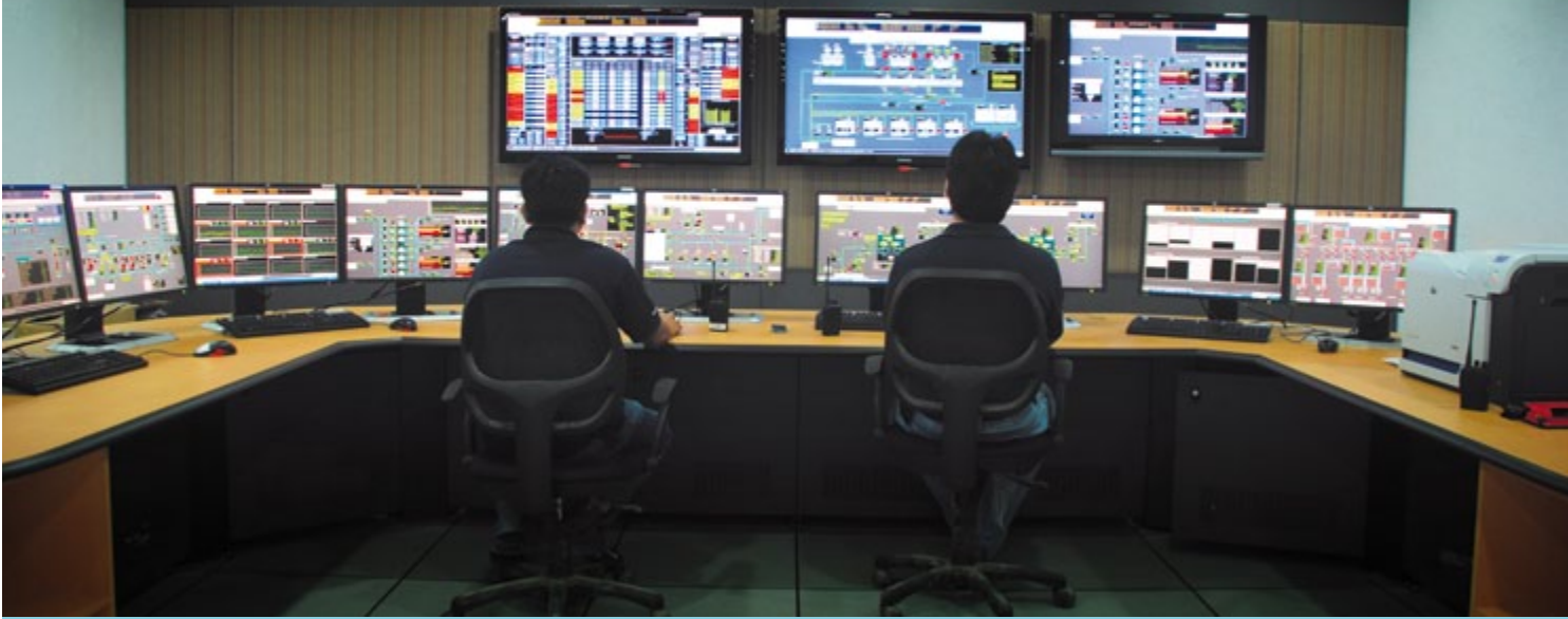
New Control Room coordinates and controls the chilled water production and its distribution to customers intake stations.
