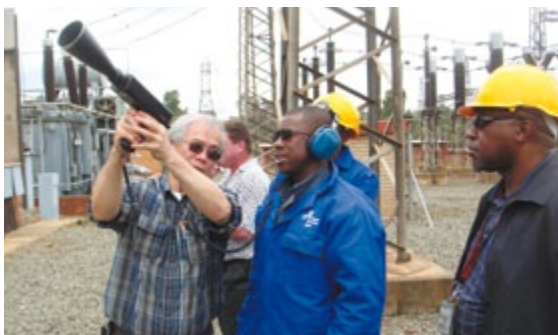
SP PowerGrid engineers conducting Condition Monitoring tests in Johannesburg, South Africa.
