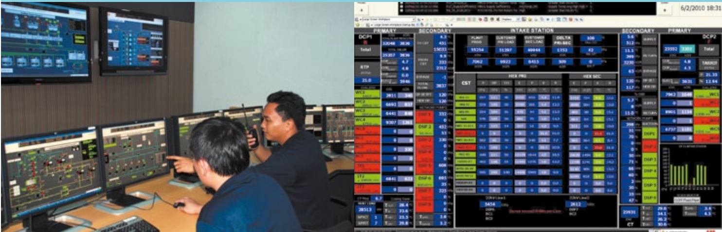
New Control Room coordinates and controls the chilled water production and its distribution to customers intake stations.
