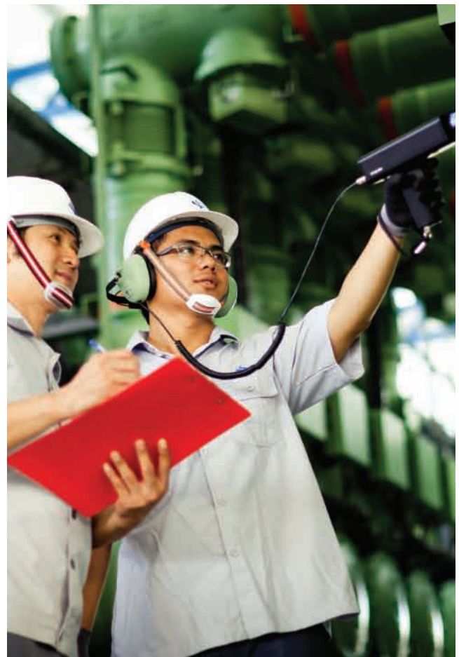
SP PowerGrid achieves excellent network performance due to its strategic use of state-of-the-art equipment and condition monitoring technology.
