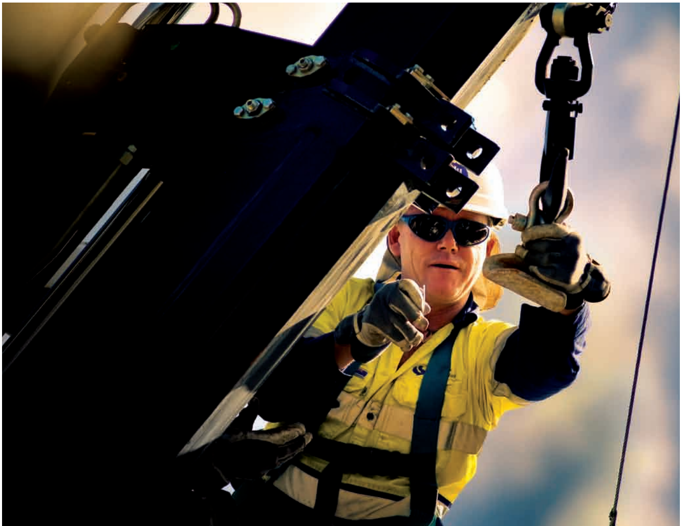
SP AusNet's electricity distribution network carries electricity from zone substations to customers in outer eastern metropolitan Melbourne and eastern Victoria.
