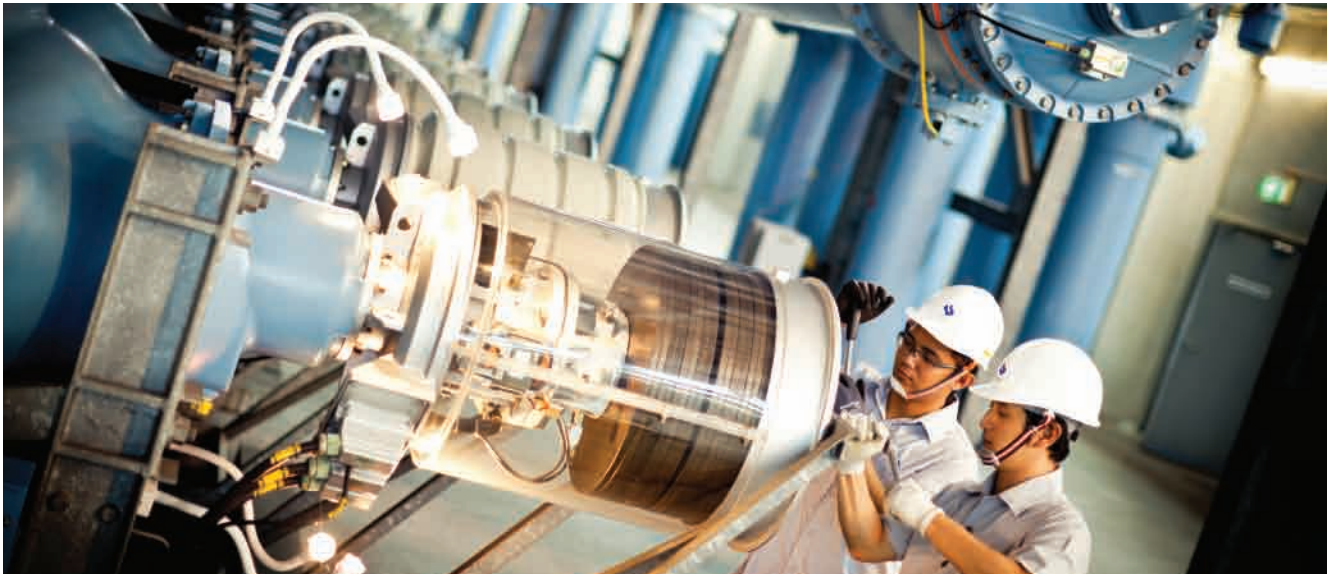
Technicians dismantling 400kV circuit breaker mechanism for maintenance.
