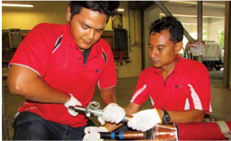
A cable-jointing workshop in progress.
