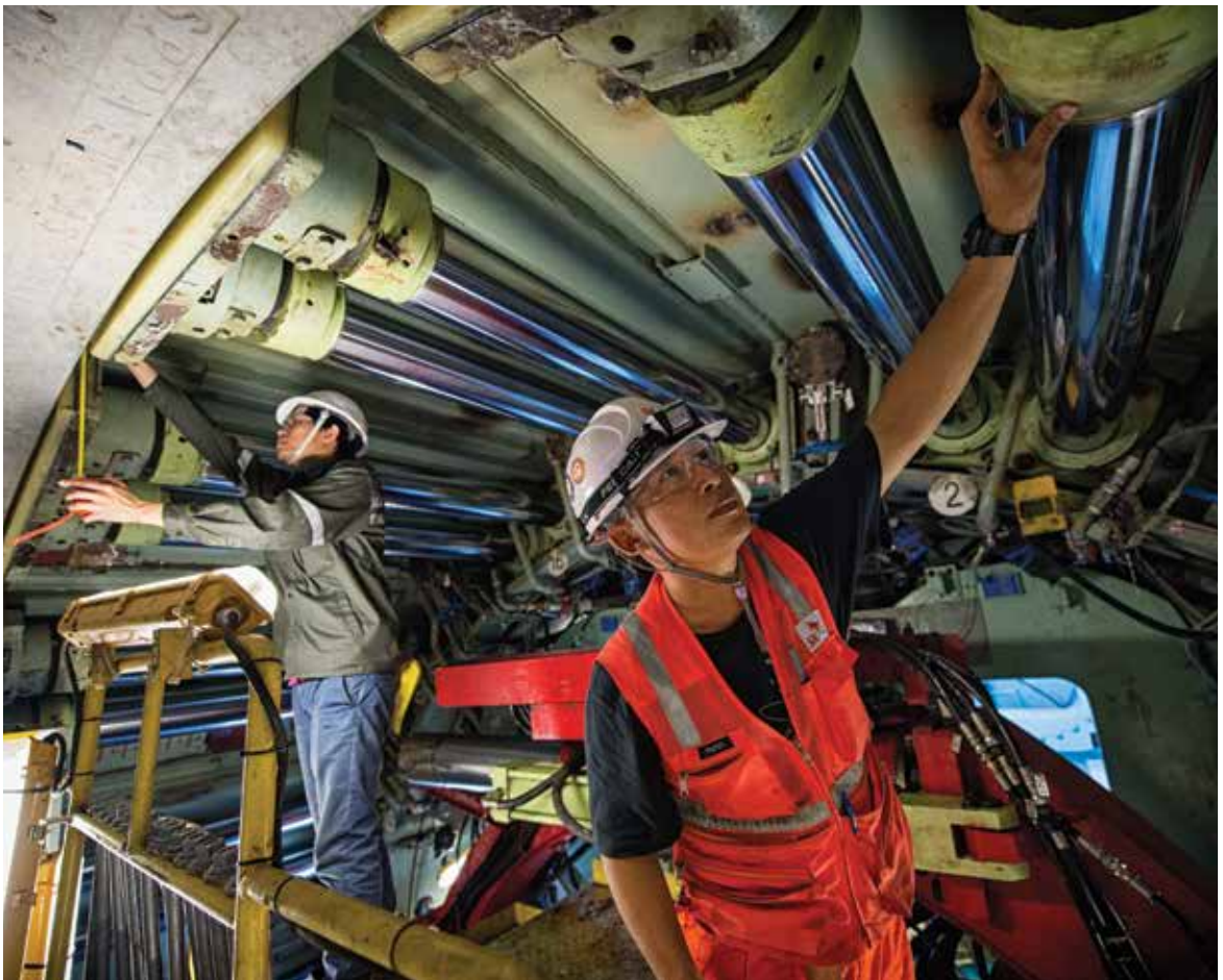
Workers at the tunnel boring machine, May Road shaft.
