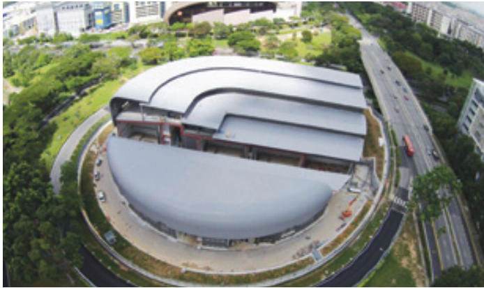
The Changi East 230kV substation meets the rapidly growing demand in Eastern Singapore
