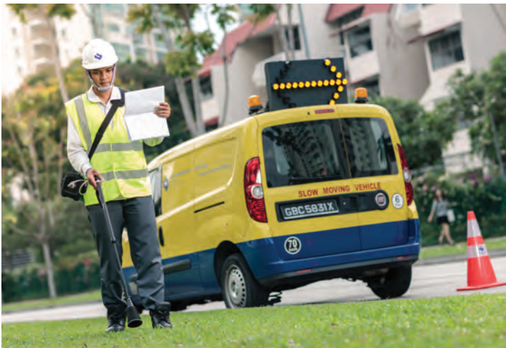
Technical Officer Mohamad Ridhwan Bin Mansor conducting a gas leak survey as part of our regular maintenance to ensure the integrity of our network.
