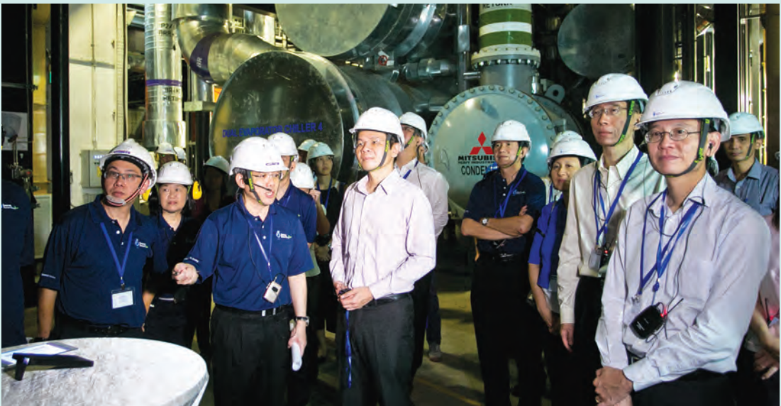
Minister for National Development Lawrence Wong toured the Singapore District Cooling's Marina Bay plant during the commissioning event on 3 March 2016.
