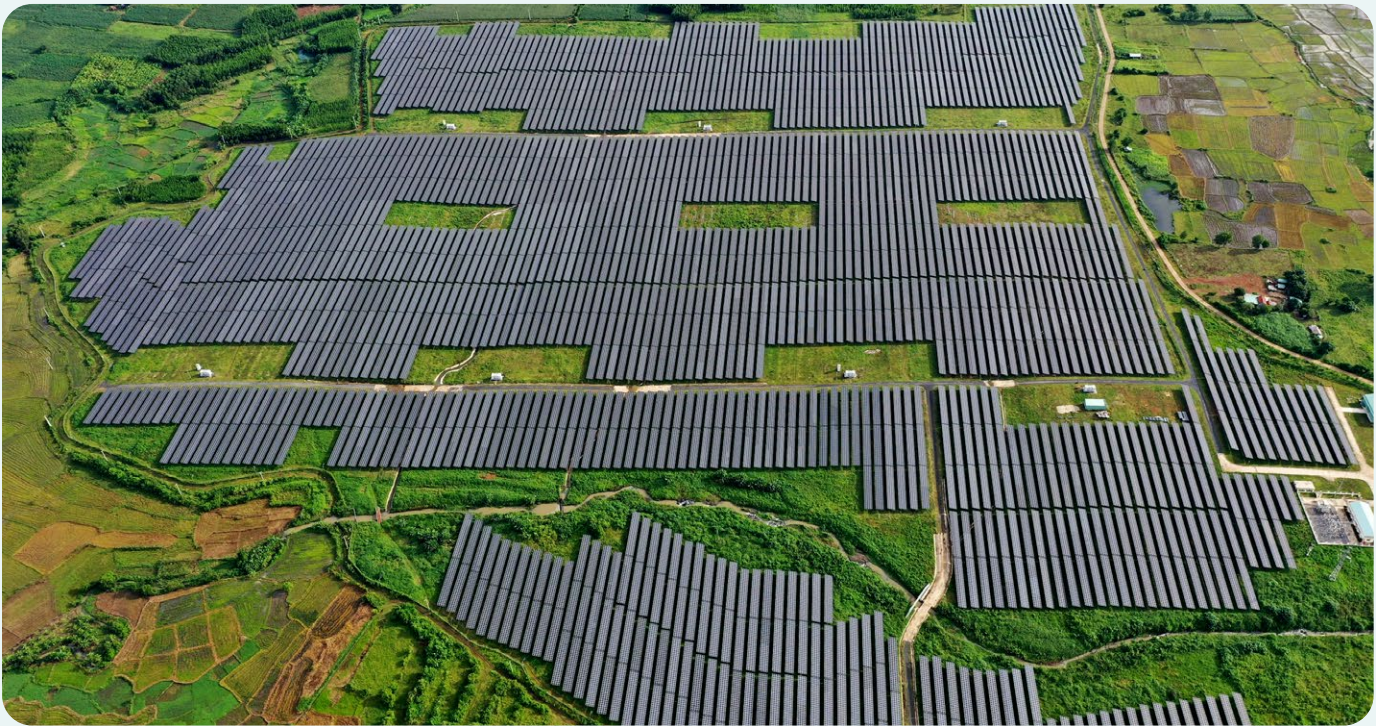
Thanh Long Phu Yen solar power plant
