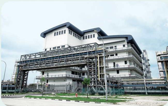
The West Jurong Island substation will be the first to have rooftop solar panels installed.
