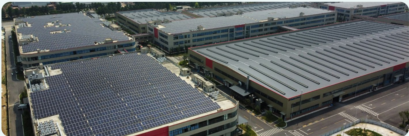
Changhong distributed (rooftop) solar project
