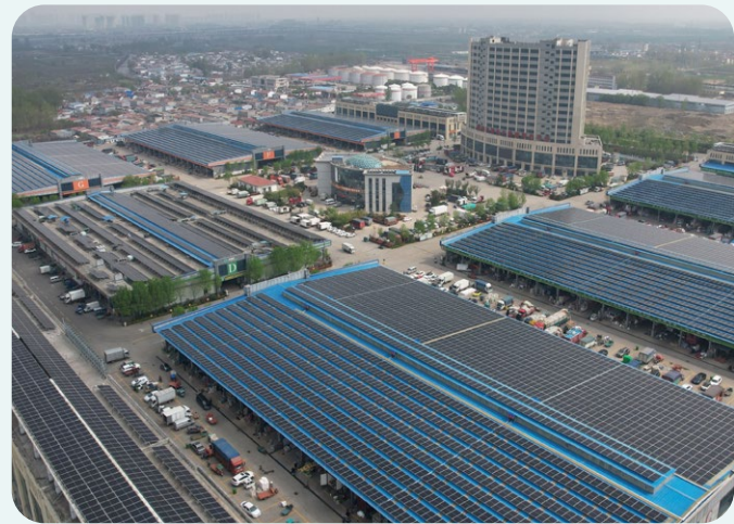
Jining distributed (rooftop) solar project
