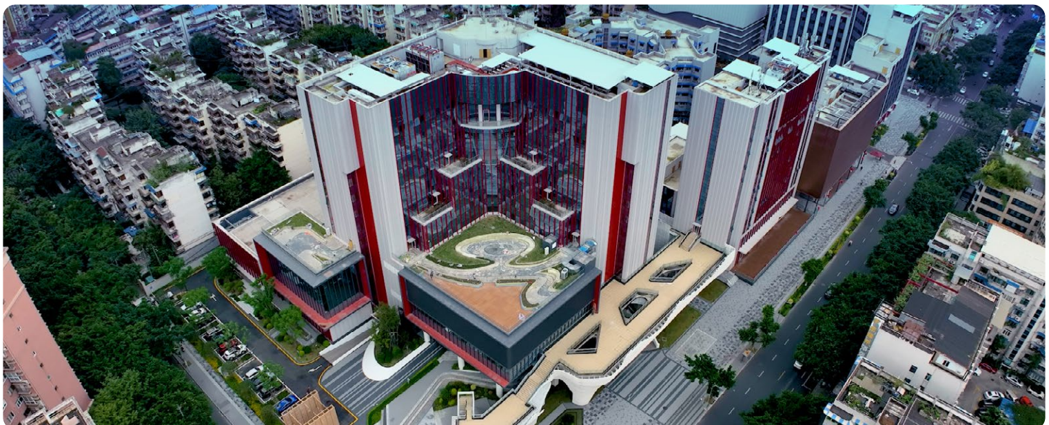
Wuhou district cooling project
